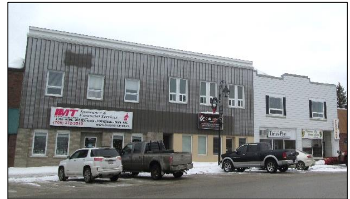
Existing commercial properties on Sixth Avenue with potential for residential in the upper storeys Image source: WSP, 2018
