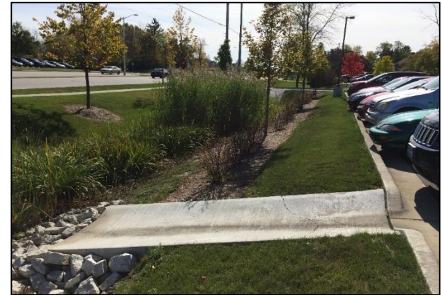
Example of a bioswale for stormwater management Image source: Aaron Volkening, Flickr
