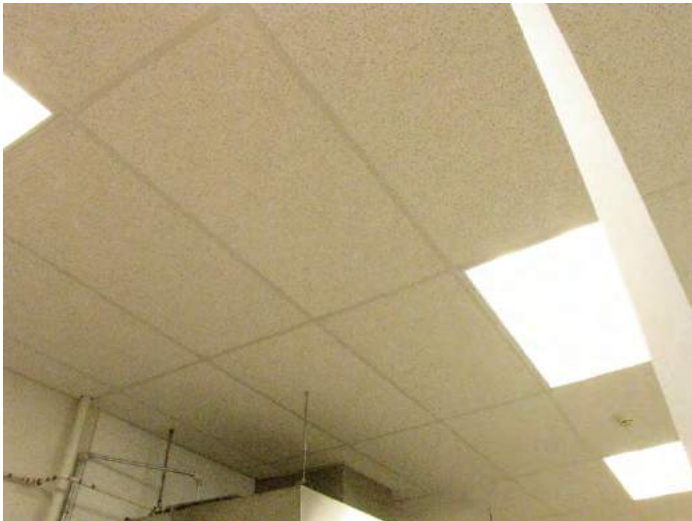
Acoustic ceiling tiles are in good condition
