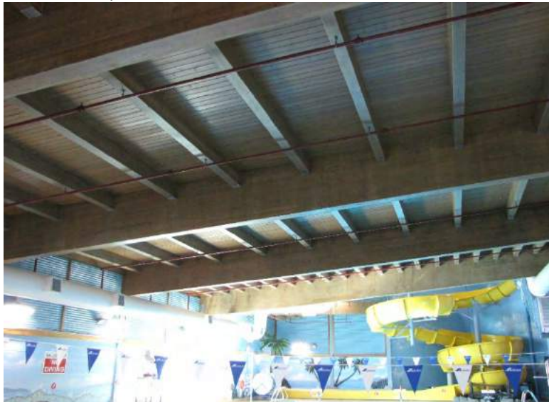
Wood beam structure and wood decking
