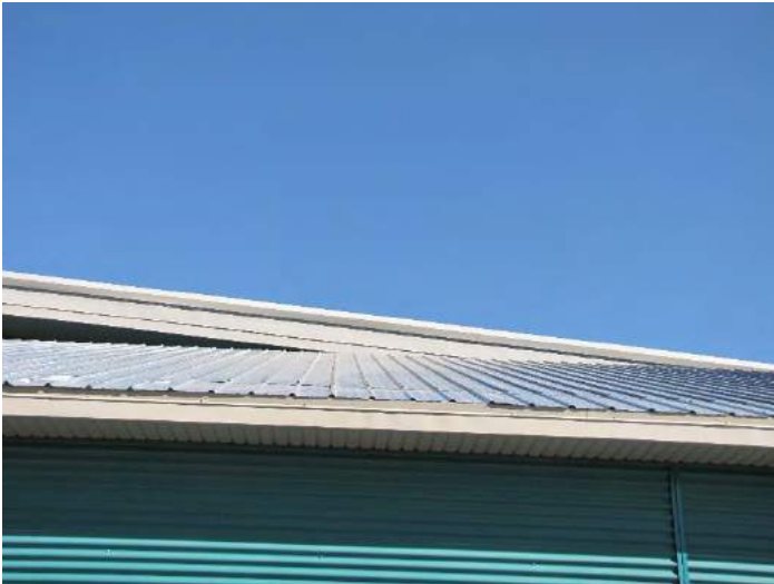
Metal roofing, snow build up is reported, as well as leaking. Exterior metal door and masonry wall, excellent condition.
