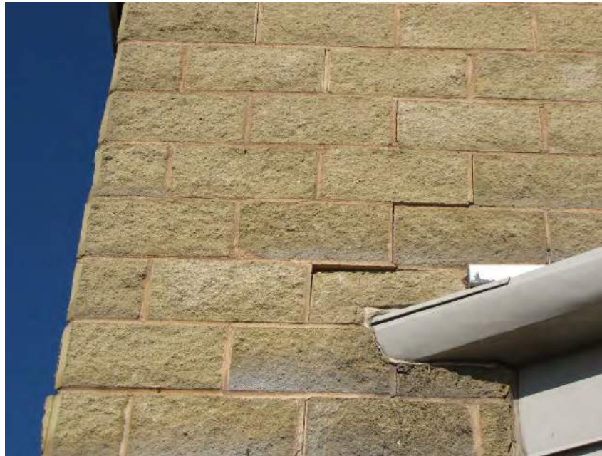
Shifting of the block and signs of water damage, likely from standing snow and water damage during freeze / thaw cycle.
